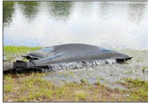
Plate 4-6 Silt bag under inspection
