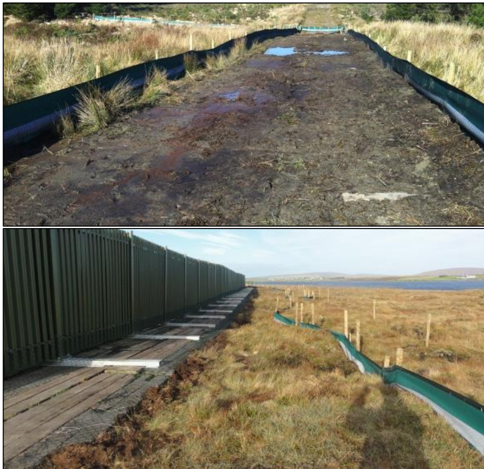
Plate 4-8 Silt Fence Details
