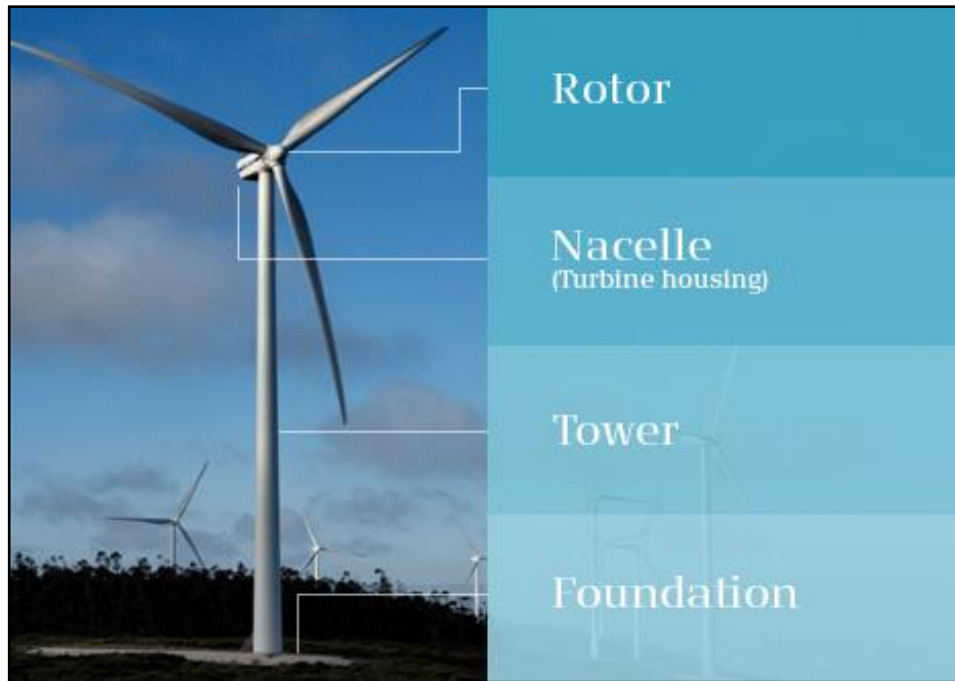
Plate 4-1 Wind turbine components
