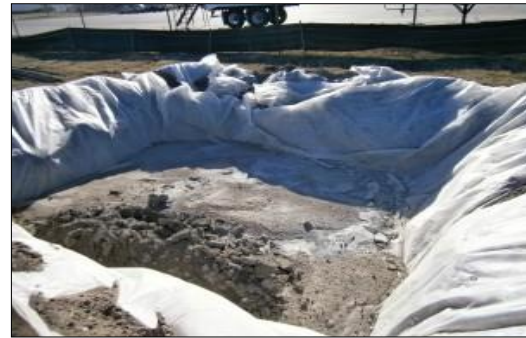
Plate 4-4 Concrete Washout Area
