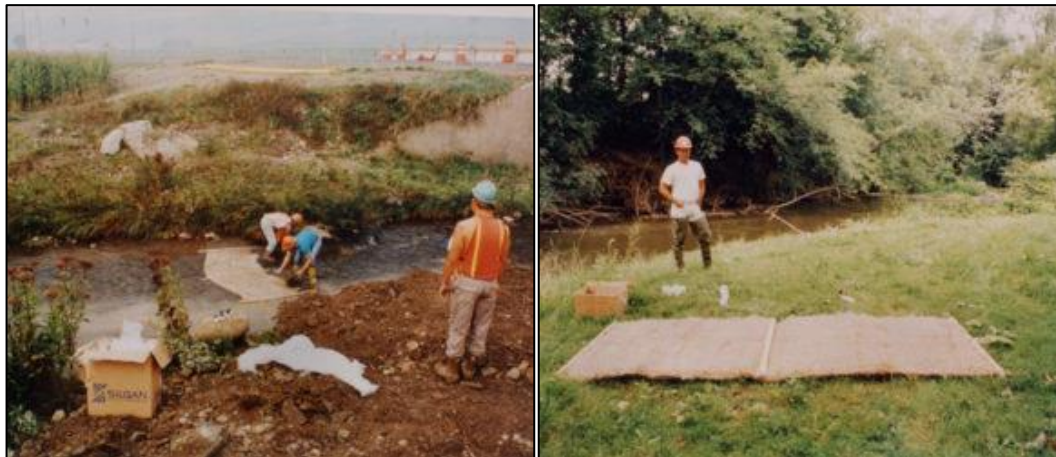
Plate 4-7 Typical Sedimat Details (Source: https://www.hy-tex.co.uk/ )
