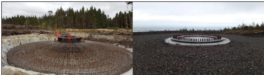
Plate 4-2 Turbine 'Anchor Cage' and finished turbine base.
