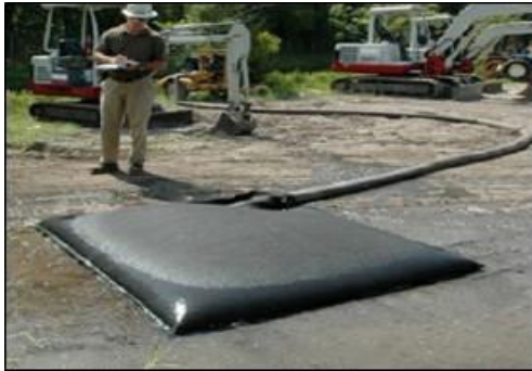
Plate 4-5 Silt Bag with water being pumped through
